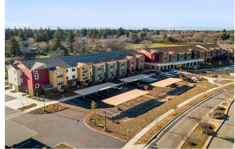
Photo courtesy of Sunseri Construction
