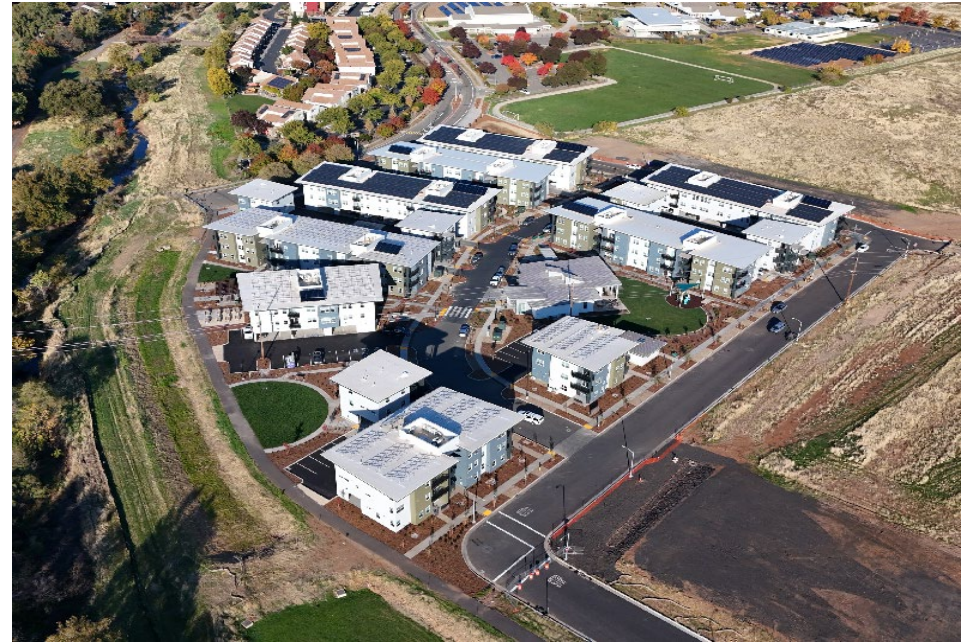
Photo courtesy of Sunseri Construction
